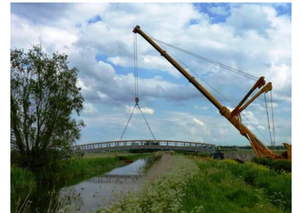
Reach bridge being lowered into place.
